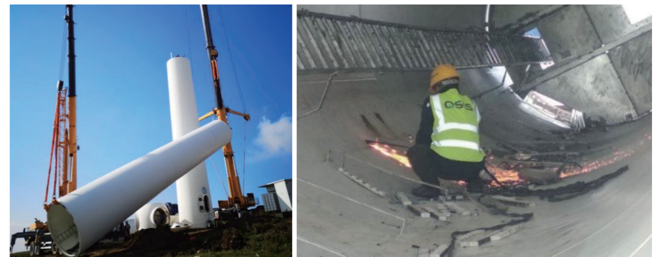
Figure 3-1: Dismantling of Wind Turbine Towers
