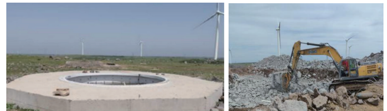
Figure 3-6: Dismantling of Wind Turbine Foundations
