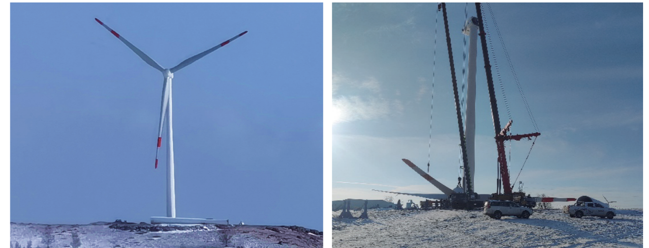
Figure 5-1 On-Site Implementation Photos
